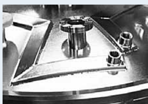
Water channel construction
